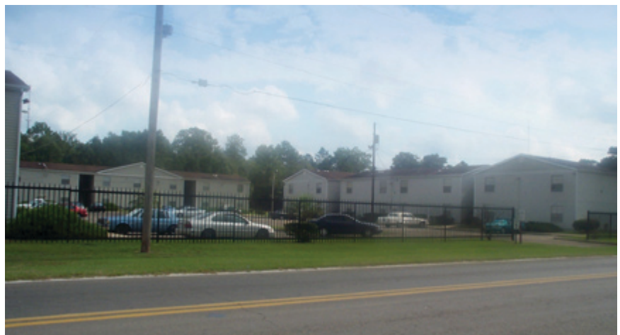
Briarwood Manor multi-family housing complex along Shelfer Road across from Oak Ridge Elementary School. Only 5% of the sector's vacant area is zoned for multi-family housing. There is agreement in the Oak Ridge Sector community to team up with the County, City, and School District to use the school for neighborhood recreational uses.
