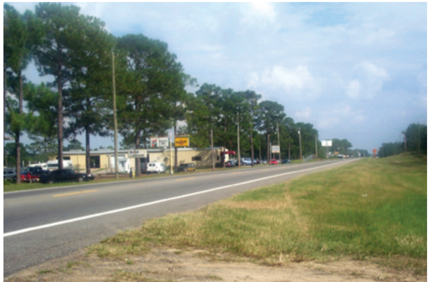
Commercial development along the north side of Capital Circle SW abuts the Apilachicola National Forest on the south side of the road.
